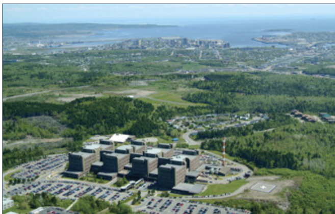
View of the Saint John Regional Hospital RDU.
